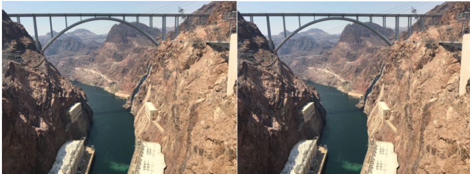
June 24, 2016: Hoover Dam Highway Bridge
